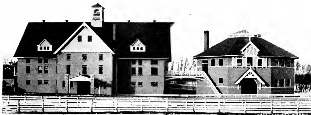
EXPERIMENT STATION BARN AND JUDGING PAVILION AT AMES, IA.
